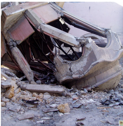
Detail of the distruction
